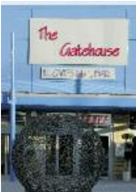
Lloyds No.1 Bar, Chichester The Kingspan KoolDuct® System purged the need for the probable introduction of secondary steel supports in this existing single storey steel frame structure, for the new suspended ceiling and major ductwork serving the new services installation.
